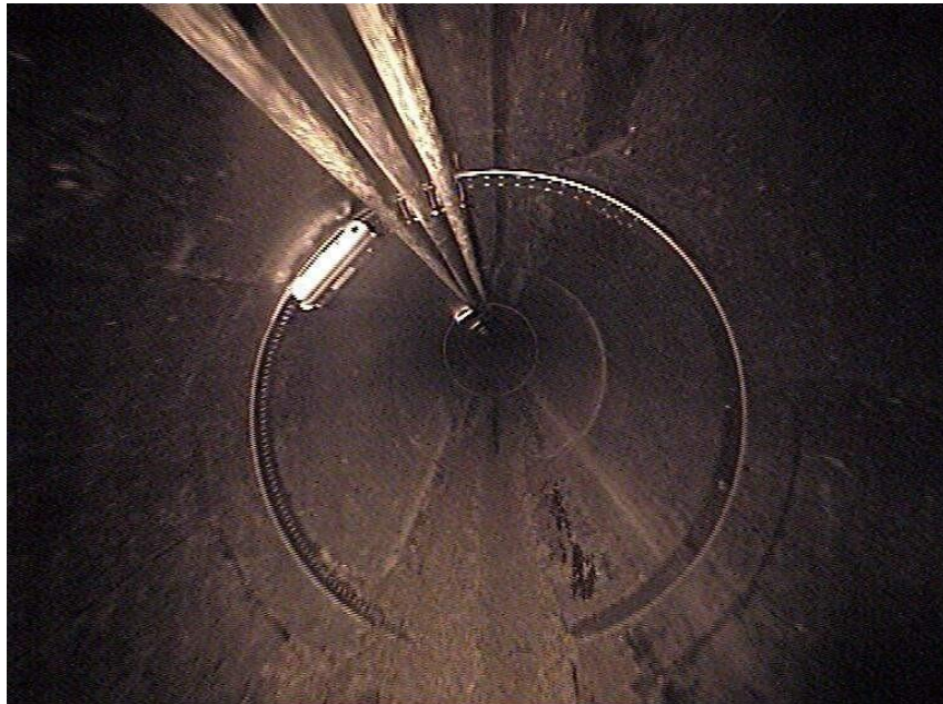
FAST-Leerrohre an Bride
